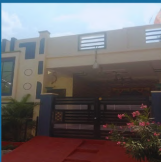
INDEPENDENT HOUSE CONSTRUCTION
